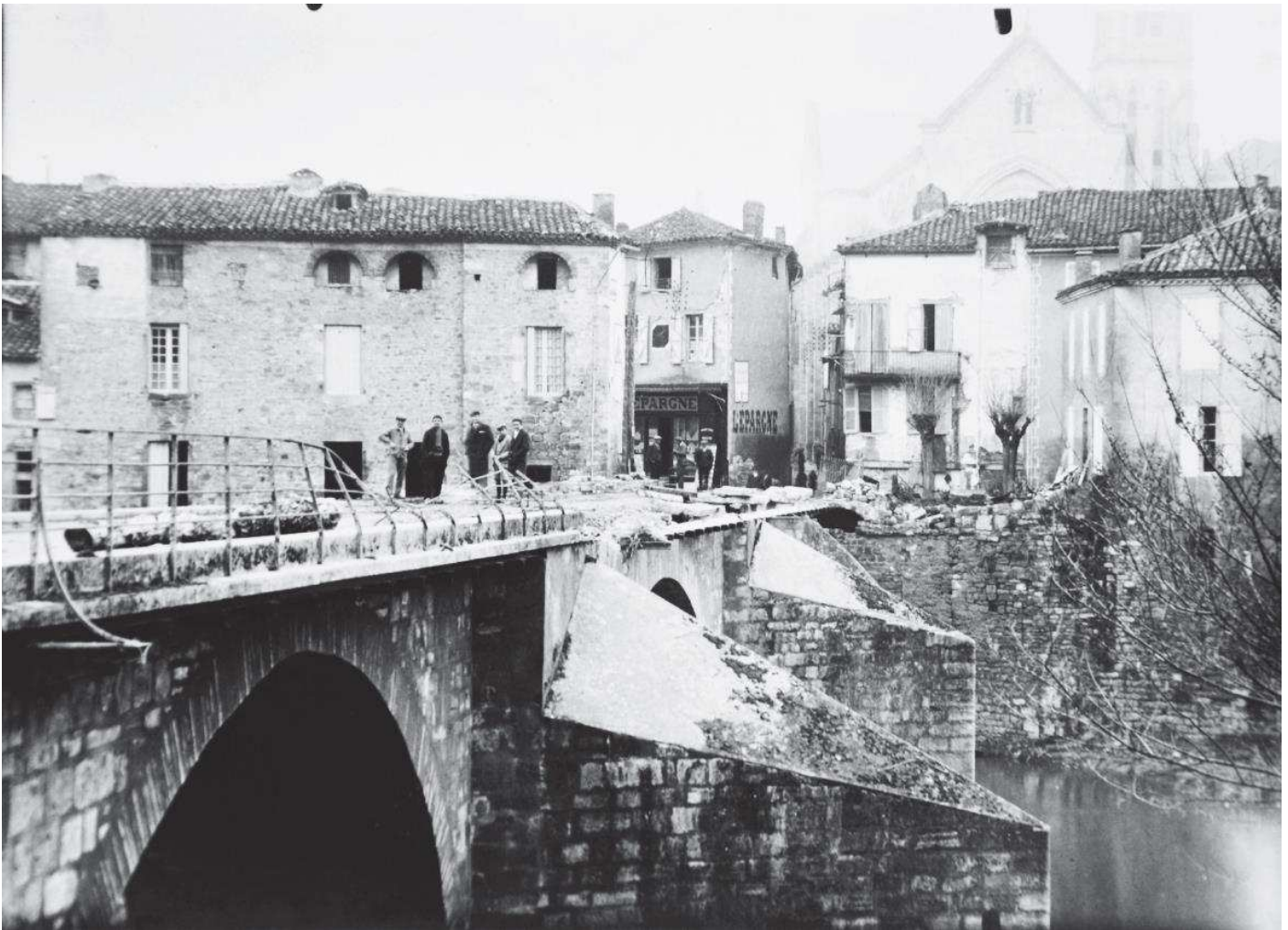
Damage to the town bridge caused by water and debris washed over it in the 1930 flood
